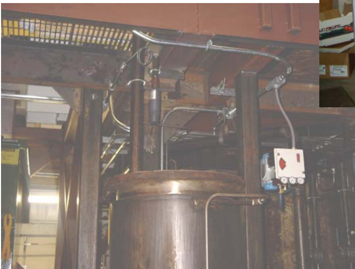
Holding Tank Ultrasonics
